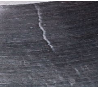
Acceptable cracking
